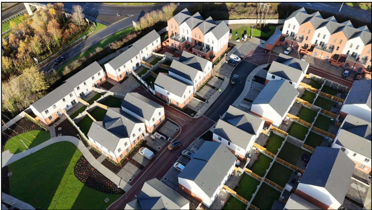
Figure 1 Drone Photograph of Gort Mell Phase 2
